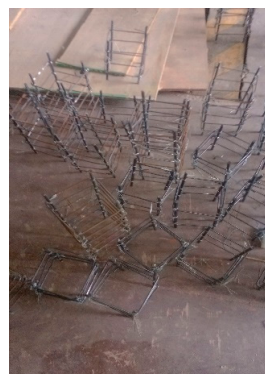
Figure 2. Assembled steel cages.
