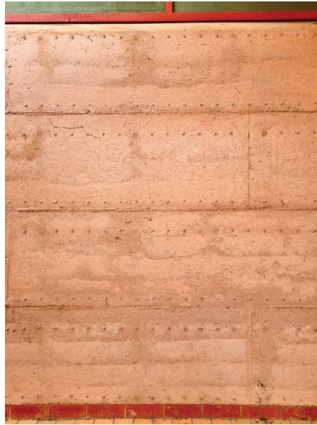
Figure 12. Section of an external wall covered by a large overhanging roof. Note the details of the recessed bolts holding the form boards as well as the sections of form boards (Bldg 762).
