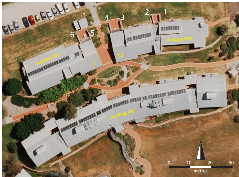
Figure 6. The School of Environmental Sciences building complex, Charles Sturt University, Thurgooona, showing the location of the buildings and the eight walls under discussion (1–6, C1, C2). Base image: Google Earth.
