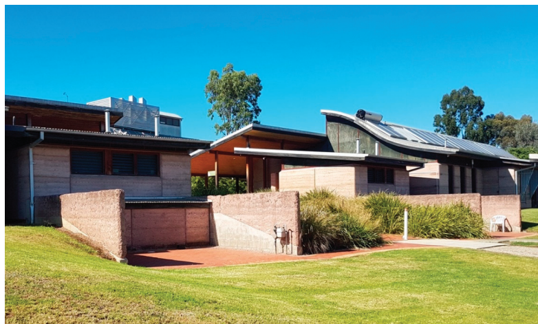
Figure 7. Uncapped pise wing walls (walls 3 to 6), as seen from the northeast. Building 761 (right) and building 762 (left).
