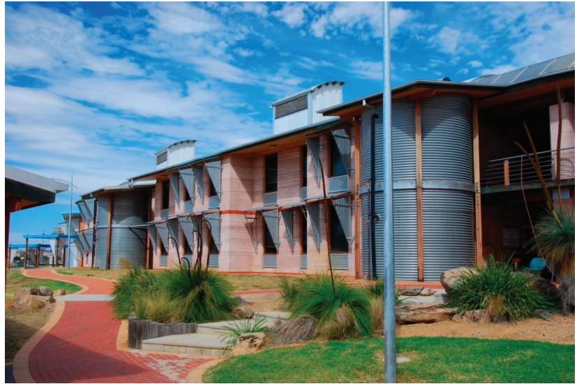
Figure 5. The eastern wing of the Environmental Sciences building (Bldg 760) as seen from northwest.
