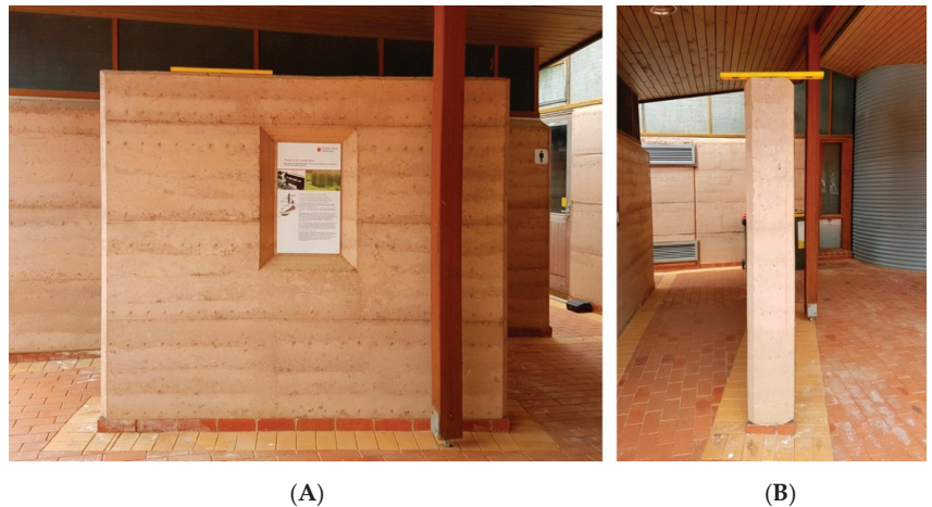
Figure 11. Uncapped, protected wall C1, screening the entrance to the external toilets of building 762: (A) frontal view seen from the south; (B) sideways view seen from the west.
