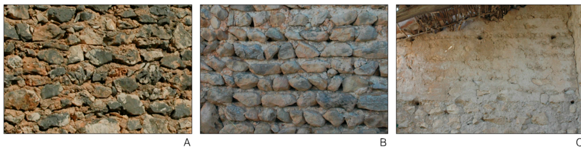
Figure 6. Compilation of detected wall fabrics. (A): Rubble stone masonry, (B): Coursed rough stone masonry (C): Tapia .
