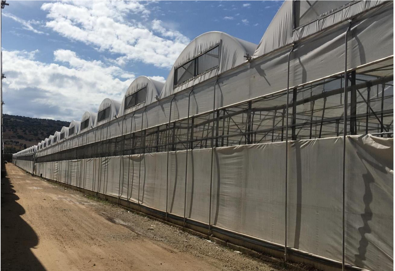
Figure S1. Characteristics of greenhouse located close to Vittoria (South-East of Sicily – Italy -36°55'19.2"N, 14°32'56.7"E) with a single module of 200 m x 35 m. The height is 6 m at the top and 4.3 m at the eaves. The greenhouses were covered with an 18-month polyethylene film with a thickness of 0.1 mm.
