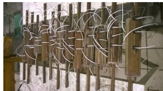
(b) Installation of strain gauges.
