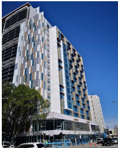
Figure 2. 18 storey modular hotel in Perth (photo by Y. Sun).
