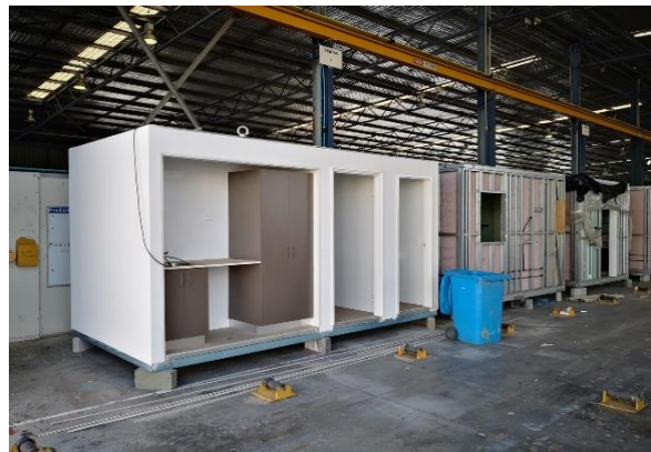
Figure 3. Module manufacture at workshop (photo by Y. Sun).
