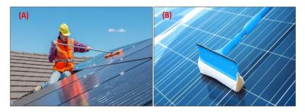
**Figure 8.** Manual cleaning process of the PV panels. (**A**) Using a soft brush with distilled water and dish soap, (**B**) using a soft brush.
