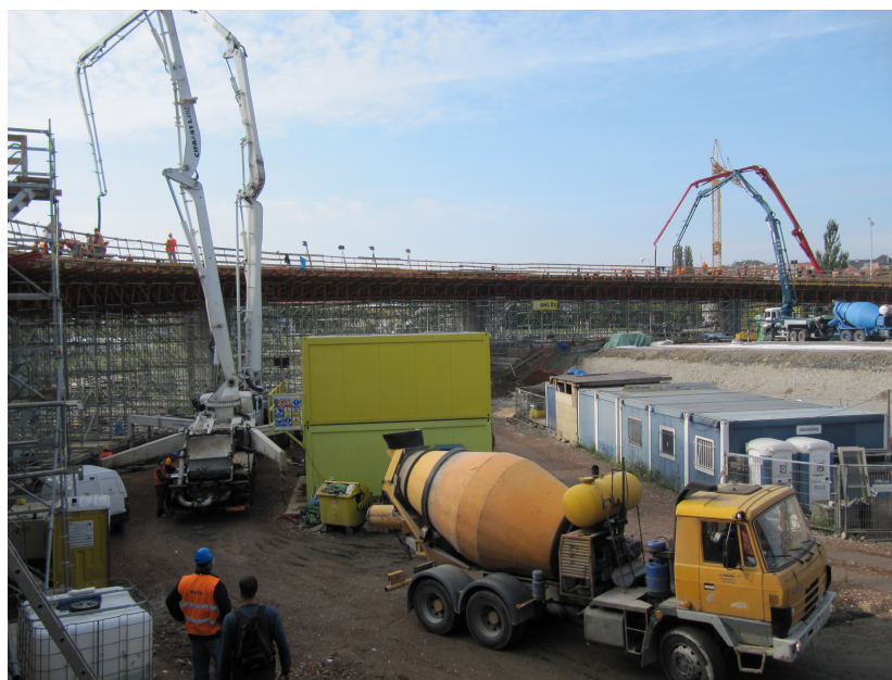
Figure 1. Bridge construction during which concrete C 30/37 XF4 was sampled.
