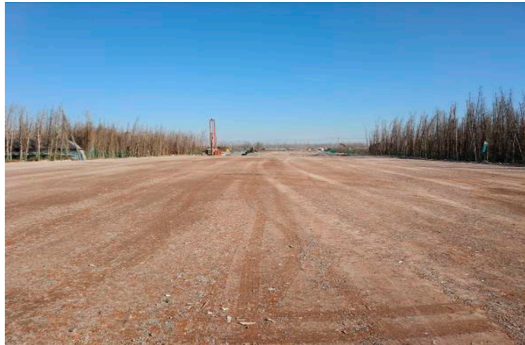
Figure 3. Highway subgrade filled with construction and demolition (C&D) materials.
