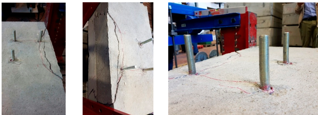
Figure 5. Specimen 3 after the shear test.
