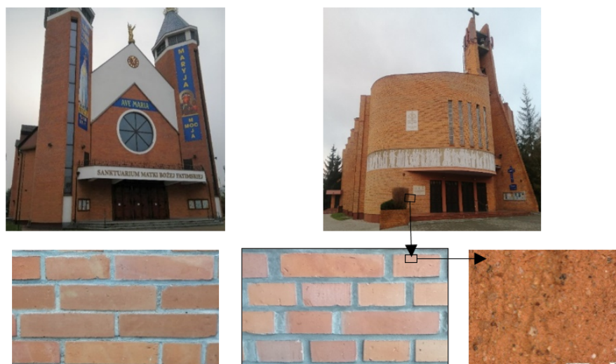
Figure 1. Religious buildings from the second half of the XX century with facing walls made of ceramic building materials with waste material additives from which the test samples were taken.
