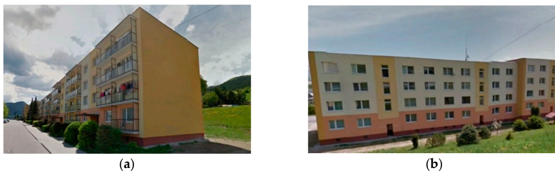
Figure 1. Residential building after the application of insulation: (a) northeast view; and (b) west view.
