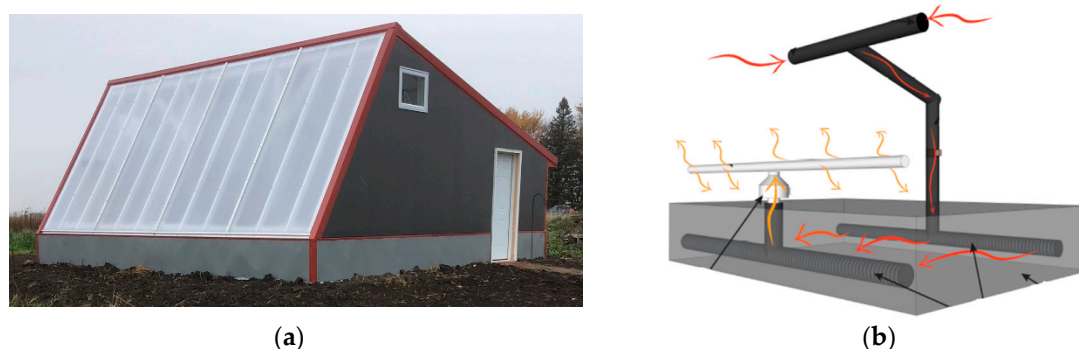
Figure 1. (a) Photo of Deep Winter Greenhouse (DWG) v2.0 at Alternative Roots Farm, Madelia, MN, taken by Greg Schweser. (b) Ductwork schematic in DWG v2.0 [8].
