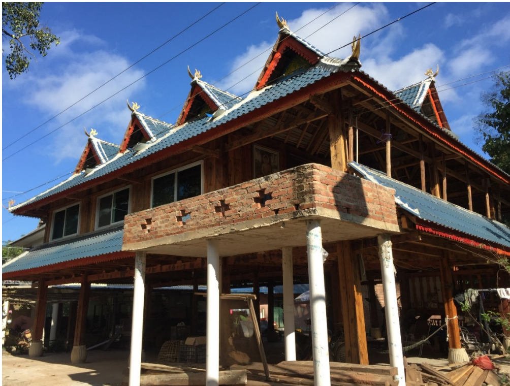
Figure 5. Hybrid style of dwelling (under construction).
