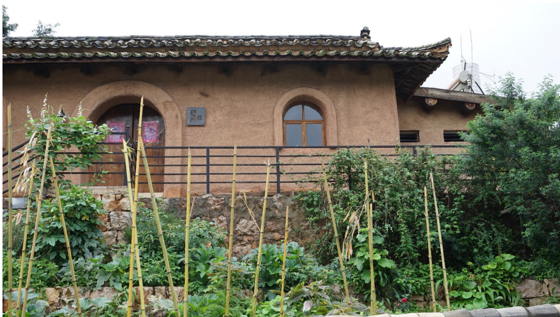
Figure 6. Damoyu—renovated mud and straw brick/adobe building.
