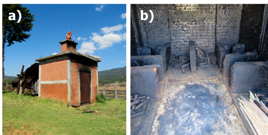
Figure 4. Exterior (a) and interior (b) view of the hand-made brick drier.
