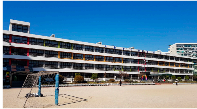
(b) School building in 2019
