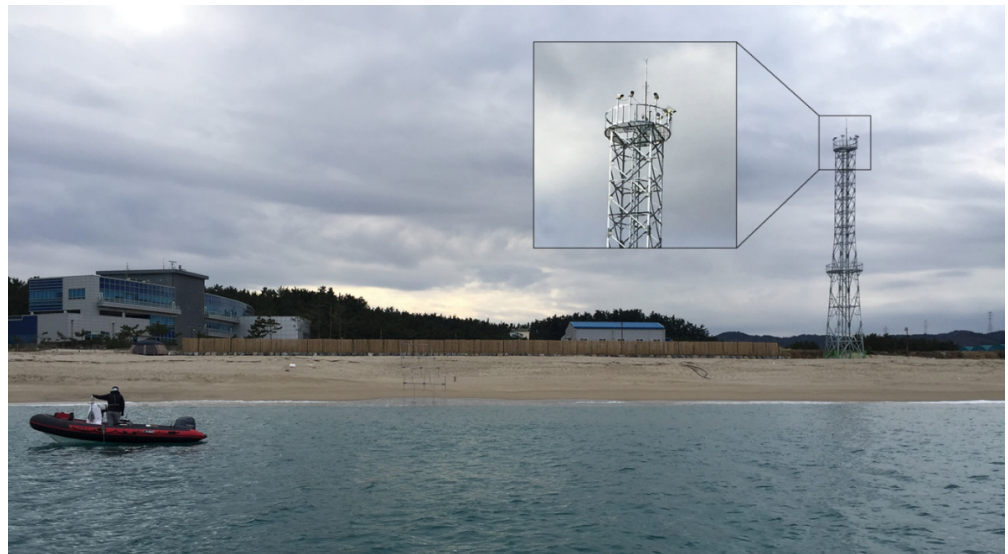
Figure 2. Photograph of the VMS with eight cameras, installed on top of a 30 m high metal tower in Hujeong Beach, Korea.
