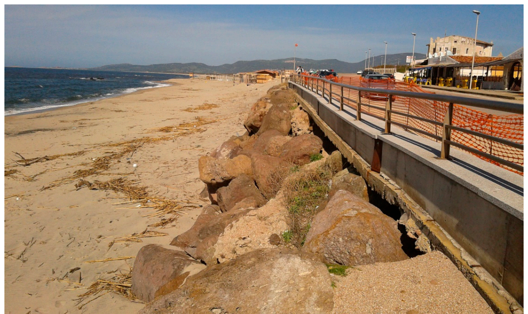
Figure 1. S. Pietro beach before interventions. The road that provided direct vehicular access to the shore had completely erased the original dune ecosystem. Photo courtesy of Maurizio Costa, Criteria s.r.l., 2013.
