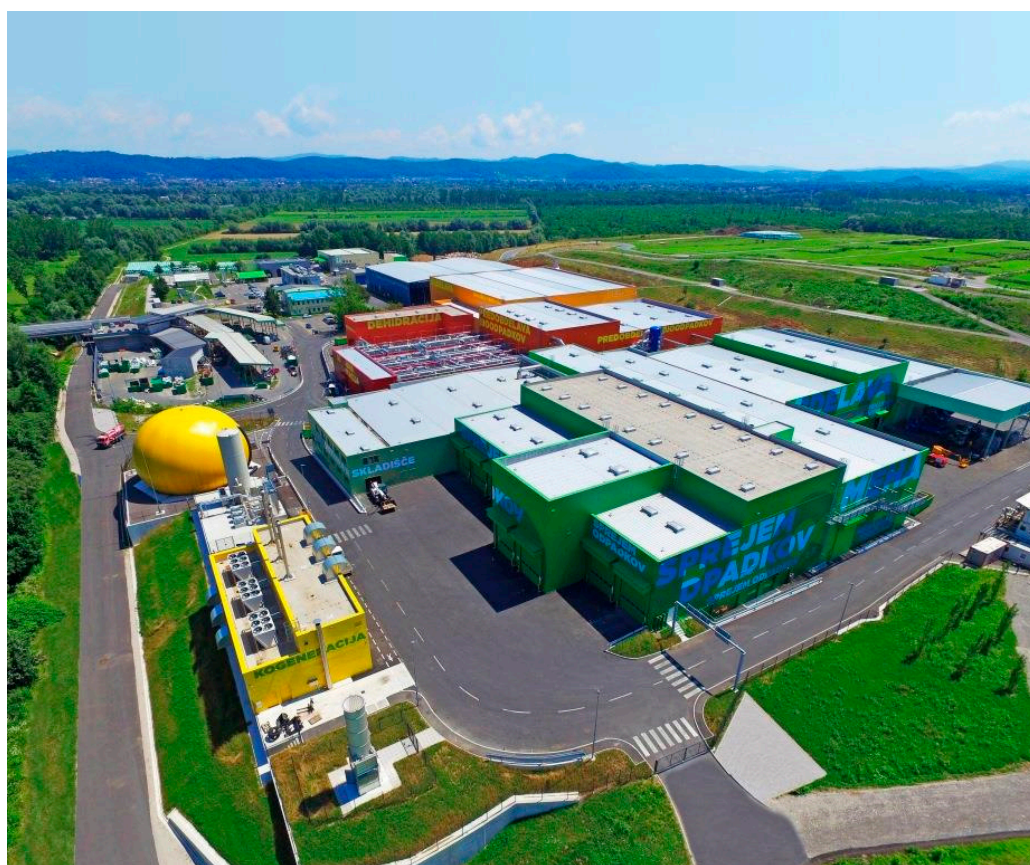
Figure 1. The Regional Waste Management Centre (RCERO) in Ljubljana (Author: SVRK/Črt Slavec, source JP VOKA SNAGA).
