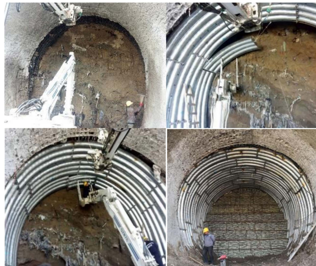
Figure 16. Assembly process of corrugated steel.
