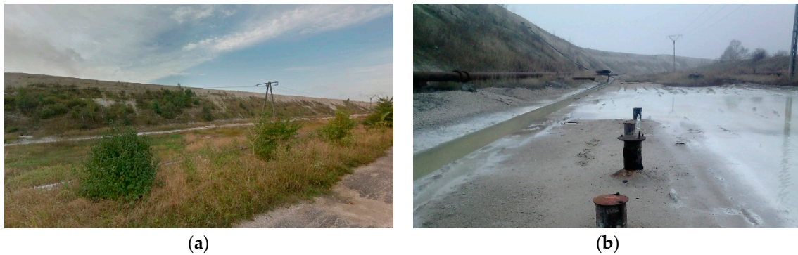
Figure 2. Heaps formed by sedimentary ponds: view from the north-east corner (a) and from the north, near piezometer W2 (b). In Figure 2b there is visible flooding area, which began to appear as the height of heaps increased. Source: own study.
