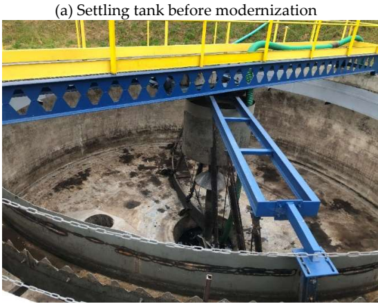
Figure S1. Reconstruction of old settling tank (a) to MBR reactor (b) Source: Own investigation
