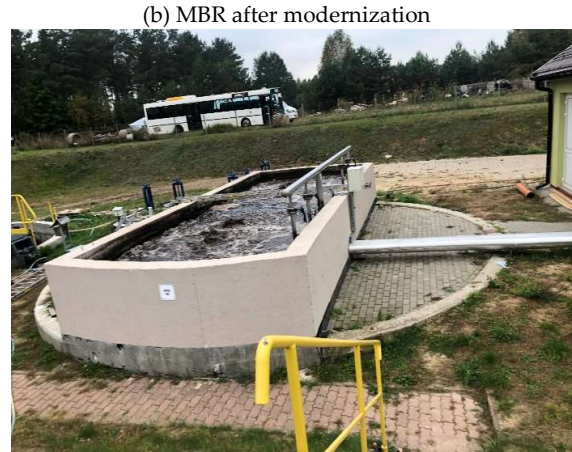
Figure S1. Reconstruction of old settling tank (a) to MBR reactor (b) Source: Own investigation
