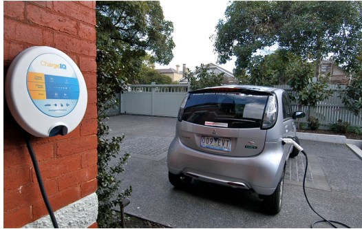
Figure 4. A DiUS Computing grid-integrated charging terminal at a participant household.
