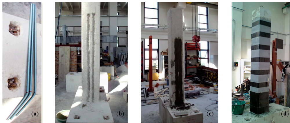
Figure 3. Strengthening procedure: layout "type A".
