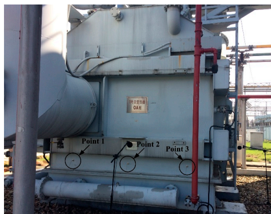
Figure 1. Locations of the vibration measurement points.
