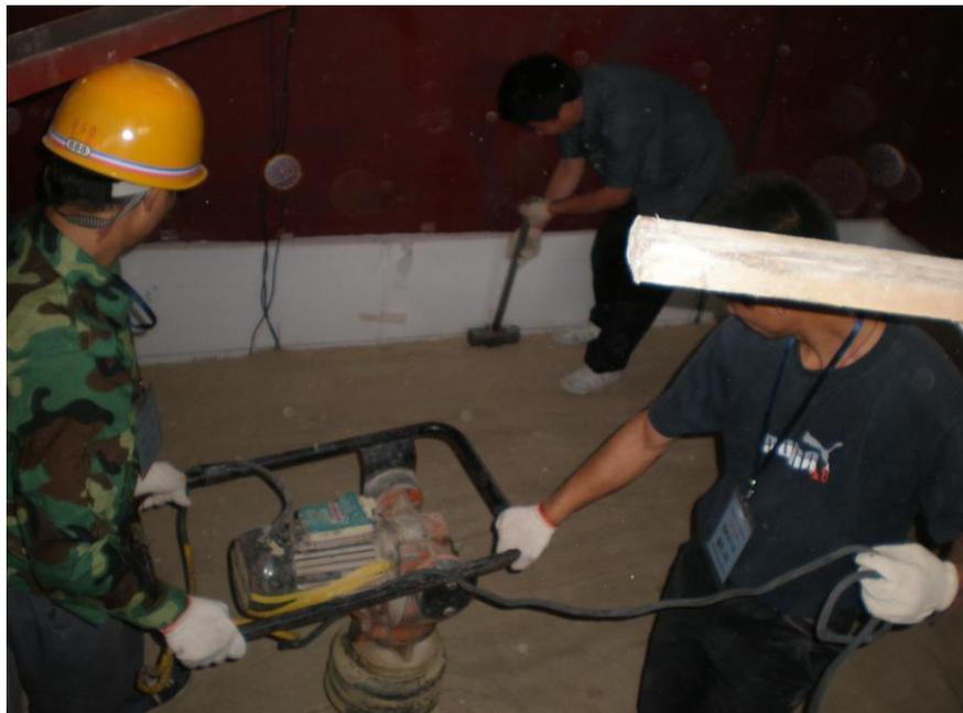
**Figure 7.** Artificial consolidation and mechanical compaction.
