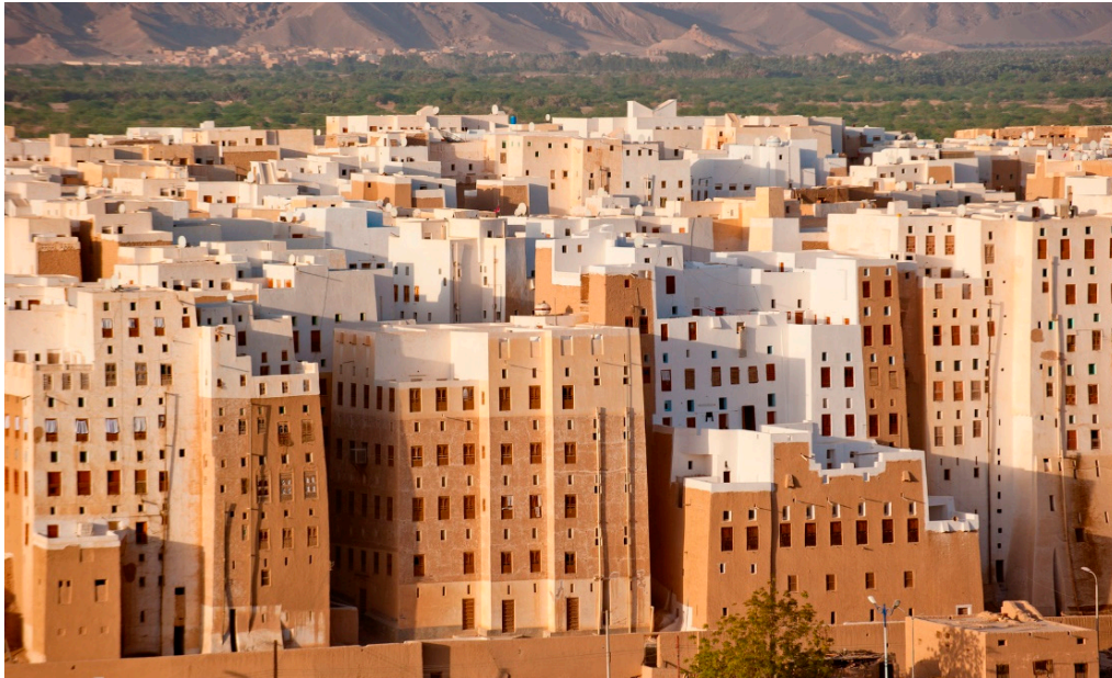
Figure 3. City of Shibam, Yemen. The city whose buildings were mostly erected with construction technologies using earth.
