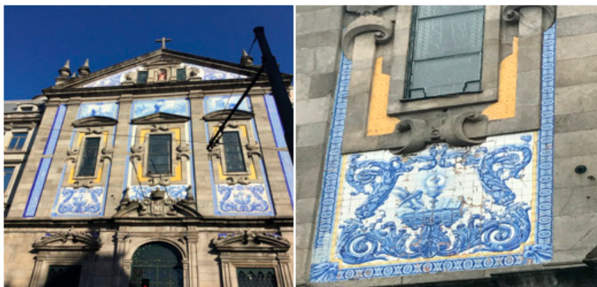
Figure 8. Facade of Igreja dos Congregados—Porto. Source: taken by author Shahrbanoo.
