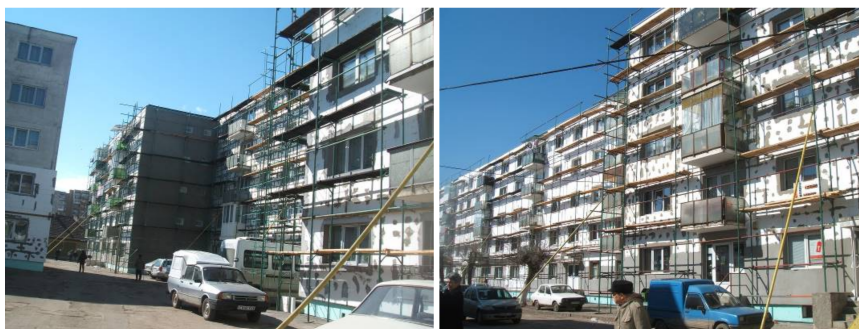
Figure 18. The apartment buildings under renovation, Prietenia compound, Sfantu Gheorghe.
