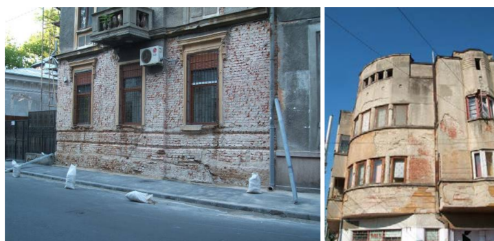
Figure 9. Low-rise and mid-rise masonry buildings, after some 80–100 years.
