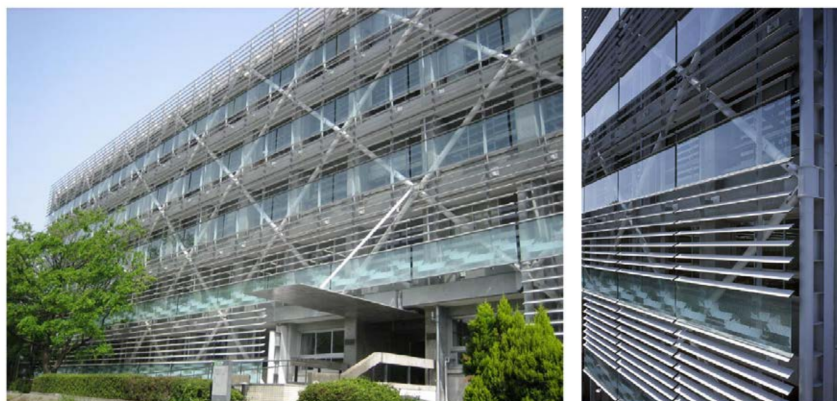
Figure 35. Midorigaoka-1st building after retrofit [103] (photographs by Mamoru Ishiguro).
