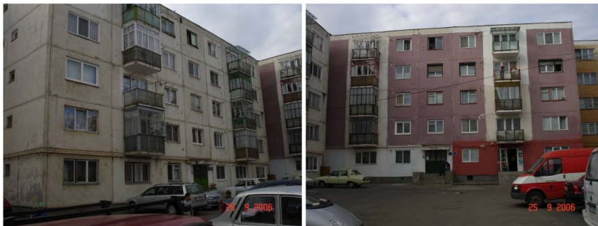
Figure 17. The apartment buildings before renovation, Prietenia compound, Sfantu Gheorghe.
