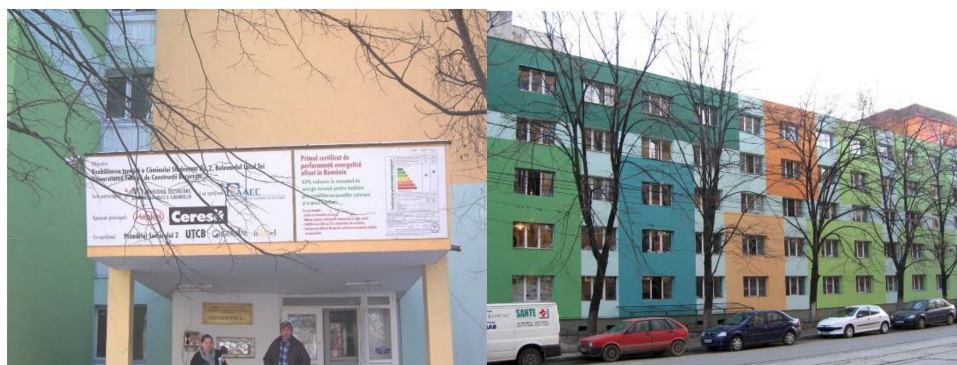
Figure 24. The UTCB Lacul Tei Students Dormitory building after energy renovation (2007). The first public building with displayed Energy Performance Certificate.
