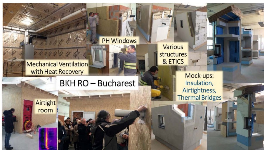
Figure 16. Practical training facility for nearly Zero Energy Building (nZEB) in the Building Knowledge Hub (Bucharest).
