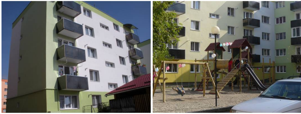
Figure 20. The apartment buildings and adjacent spaces, including playing grounds for children, at the end of renovation, Prietenia compound, Sfantu Gheorghe.
