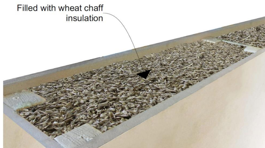
Figure 2. Filling the panel envelope of MDF board and wooden studs with dried wheat chaff insulation.
