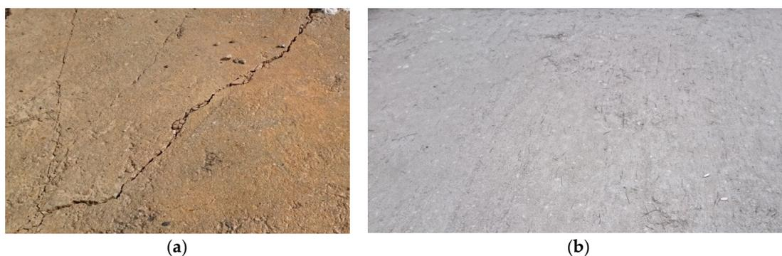
**Figure 2.** Visual aspect of the slabs after three years of service: (a) steel mesh reinforced concrete slab; (b) polyolefin fibre reinforced concrete slab.
