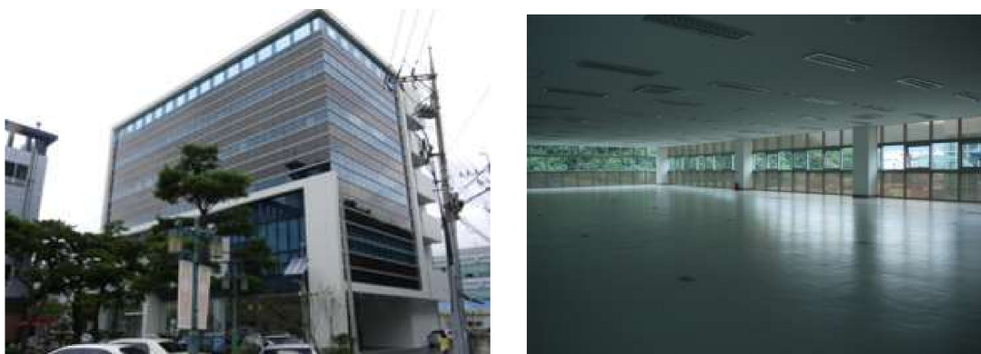
Figure 1. Outer and inner surfaces of an office building using amorphous (a-Si) building-integrated photovoltaic (BIPV) windows.
