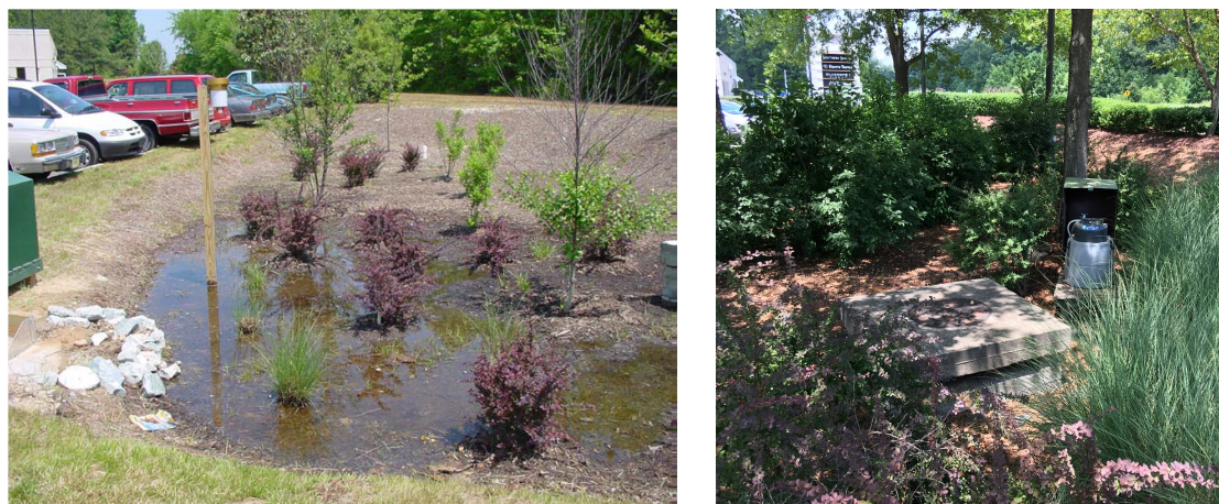
Figure 1. Bioretention cell during initial monitoring period (left) and return monitoring period (right).
