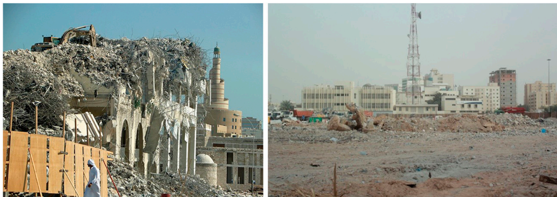
Figure 2. Demolition work affecting the vernacular al-Musheireb area in historic Doha.
