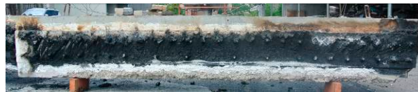
(c) Beam surface after fire
